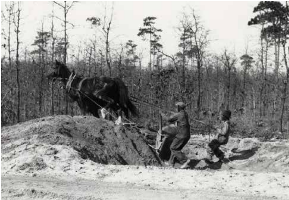
A vintage style of bunker creation in evidence at Pine Needles, North Carolina
