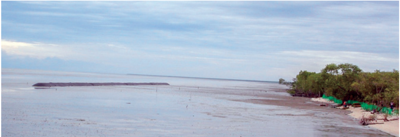
The geotube breakwaters constructed at the beach of D' Muara Marine Park Resort (before planting)
