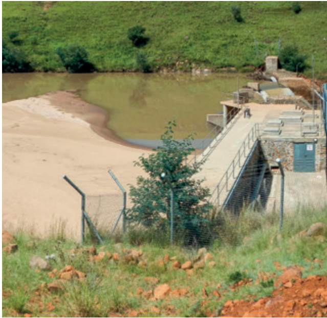
The silted-up dam at Mount Fletcher
