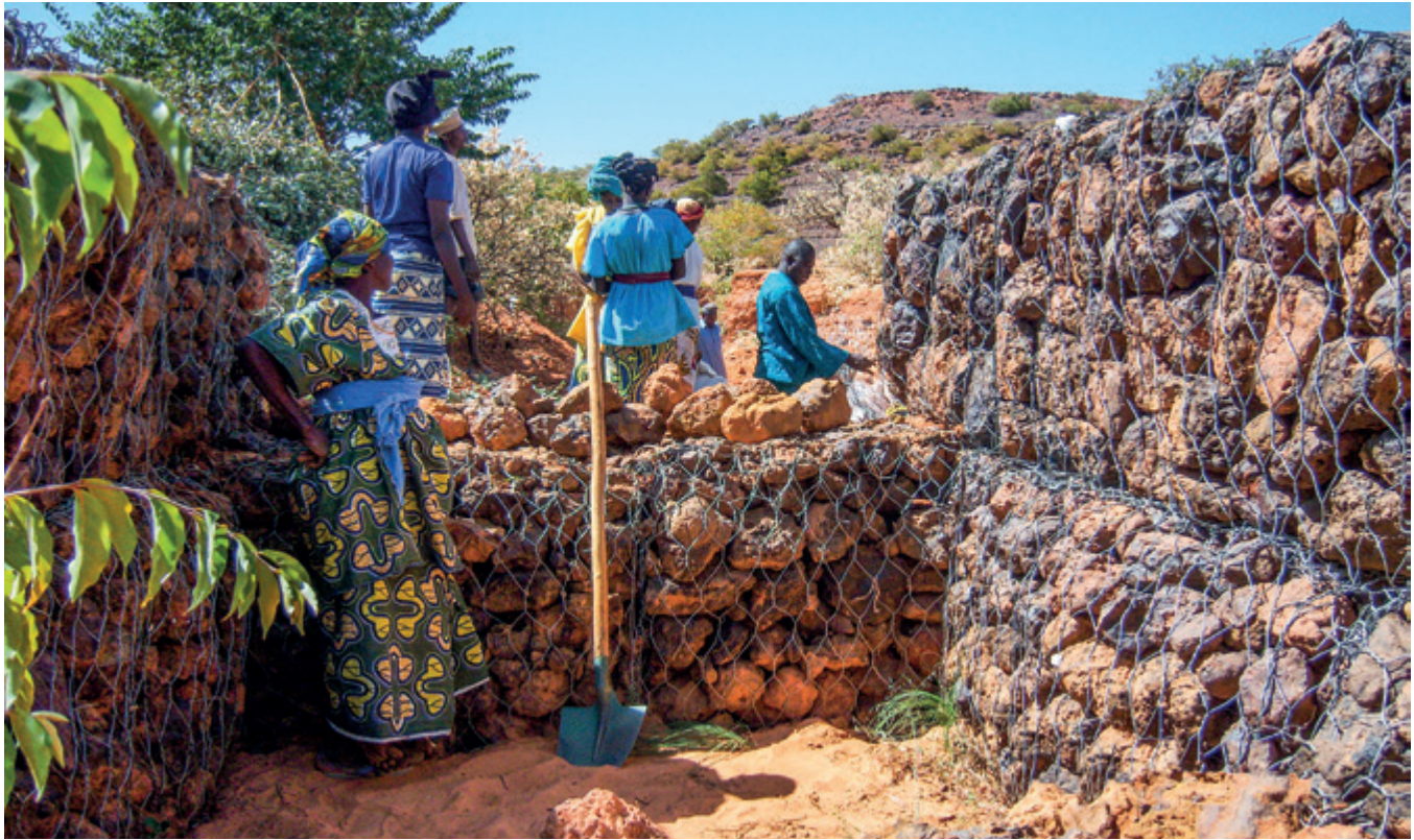
Thresholds of gabion and dry stone in the Tillabery region, Niger
