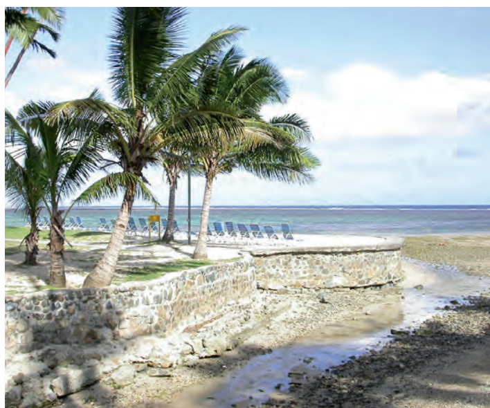
Coastal erosion and sea wall protection on a beach in Fiji
