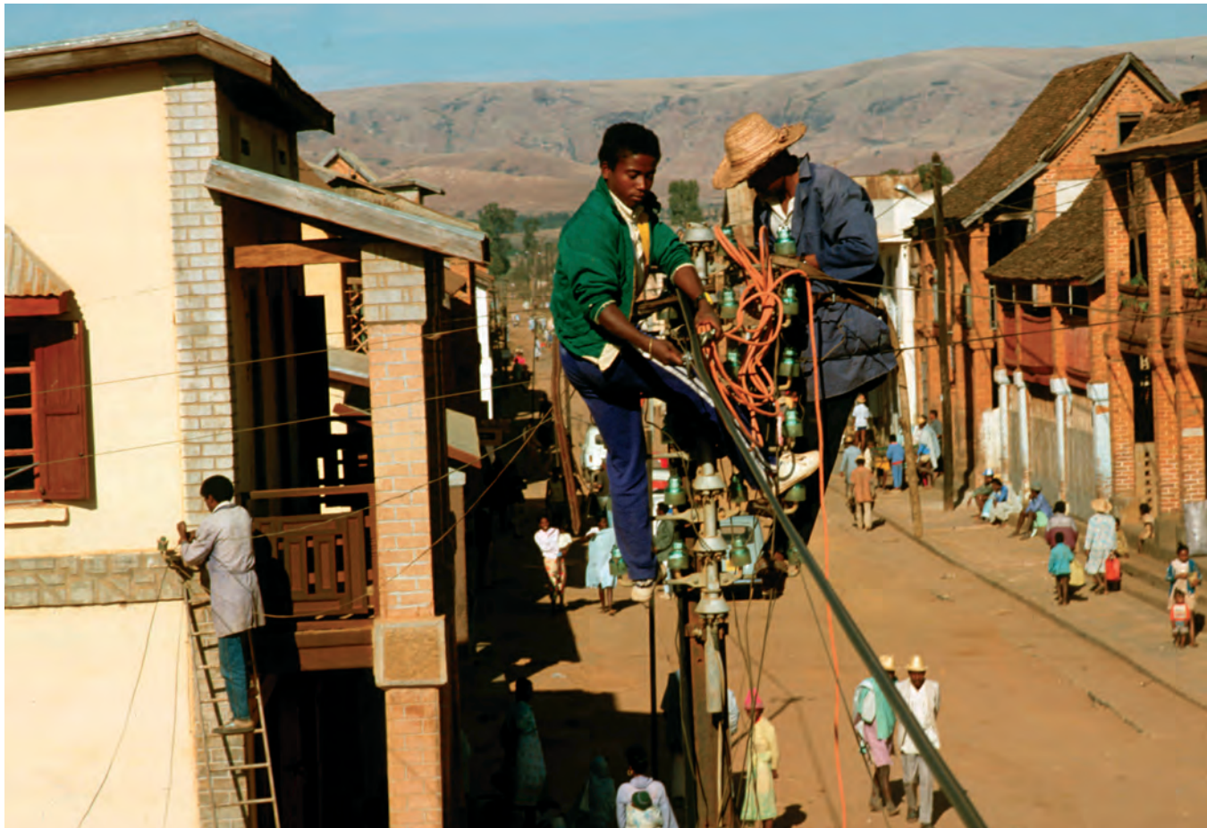
Installing a new aerial telephone line at Ithosy
