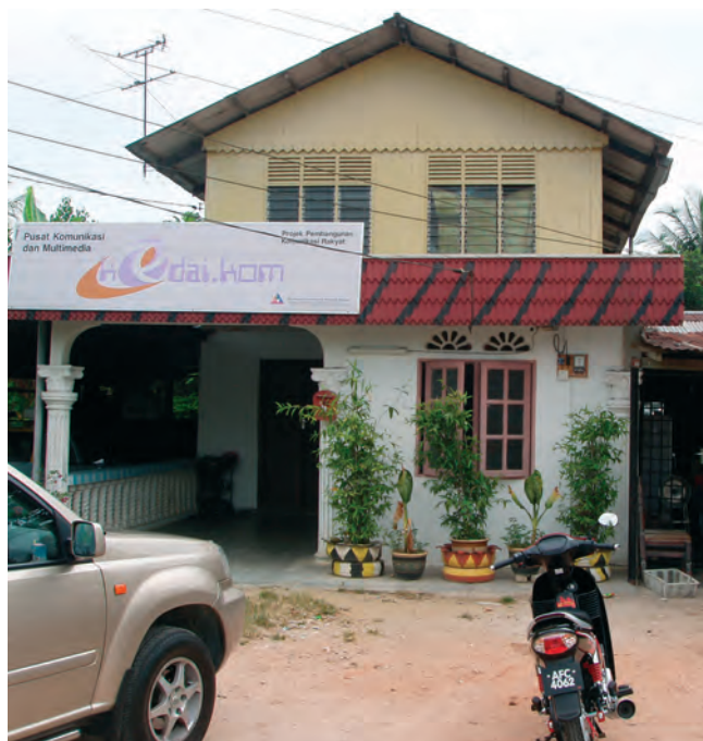
Exterior view of the CCDP site
