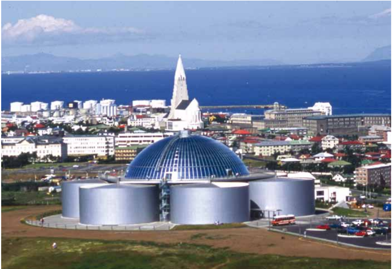
Geothermal wells piping in hot water to reservoir tanks above Reykjavik
