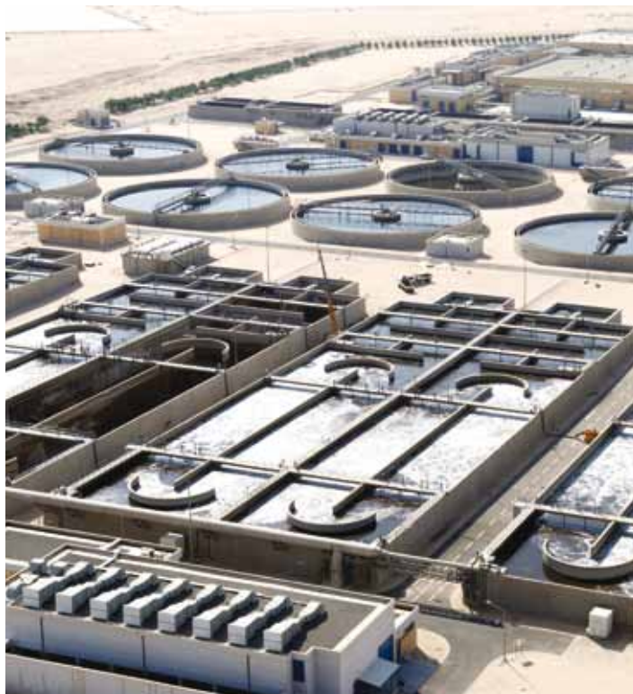
Aeration tanks and secondary clarifiers
