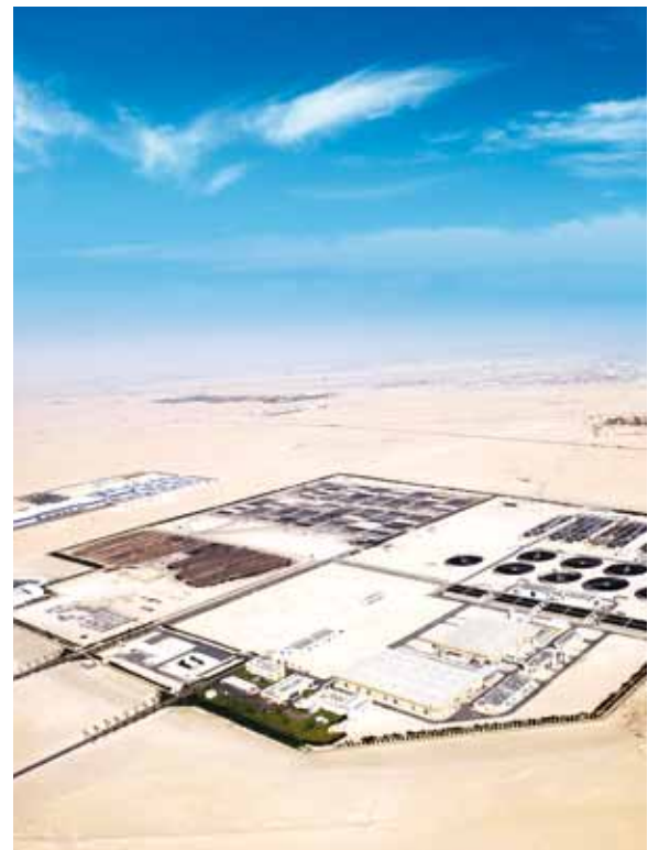
Aerial view for Sulaiybiya Plant
