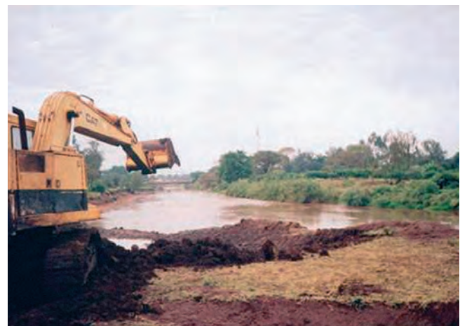
Widening the Nyando river
