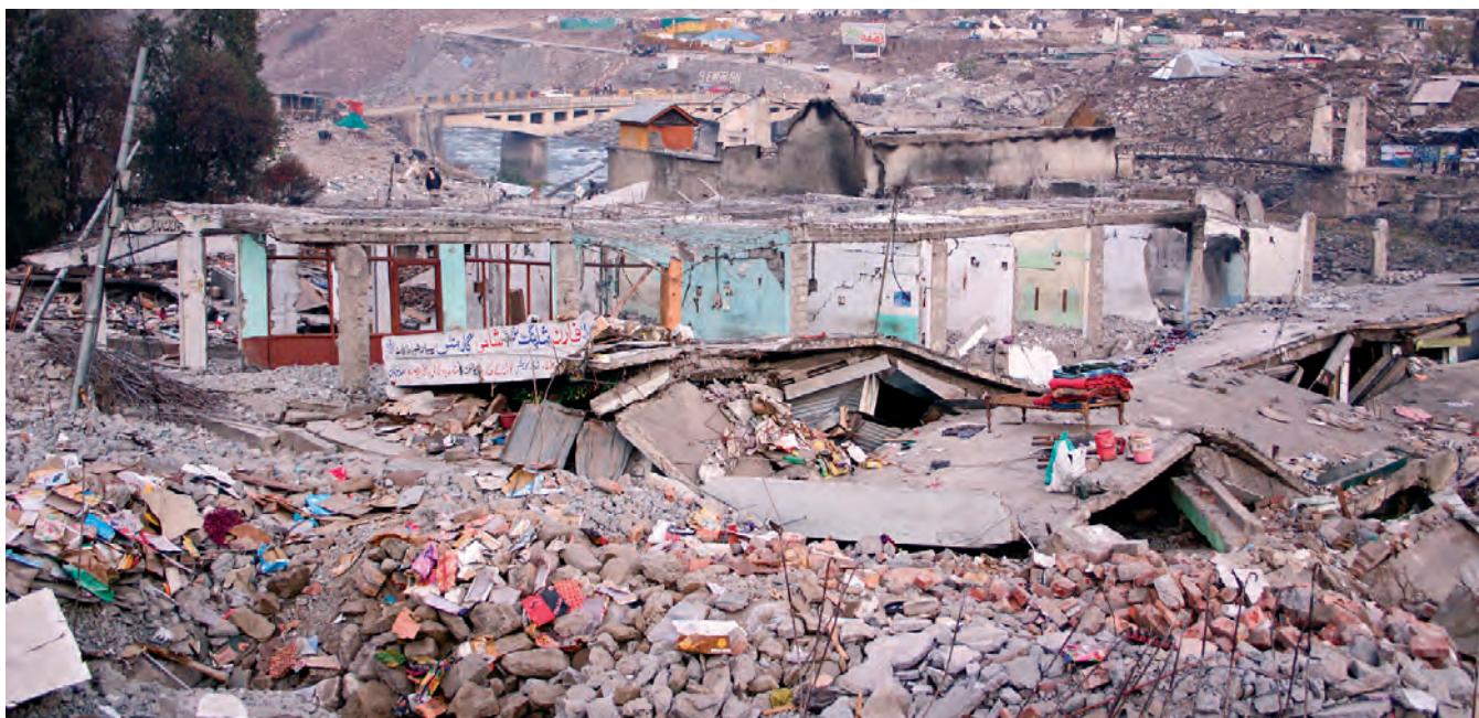
Retrofitting requires a thorough understanding of a structure's potential weaknesses
