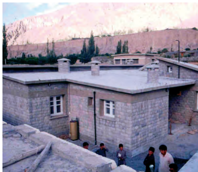
A typical seismic-resistant rural health centre
