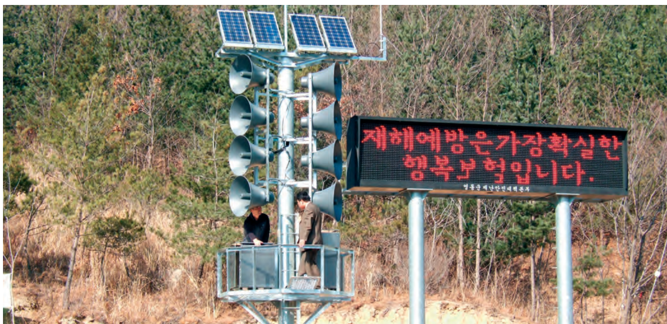
An electronic bulletin board and warning siren
