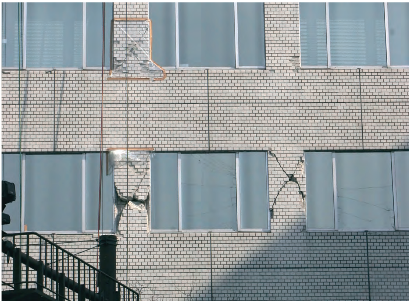
Guidelines have been developed to incorporate seismic safety into all classes of building
