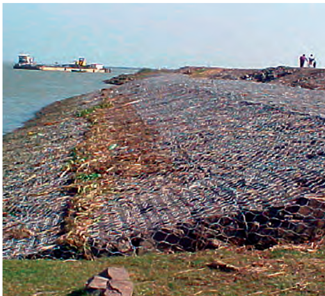
Boulder-crate technology reinforces an embankment
