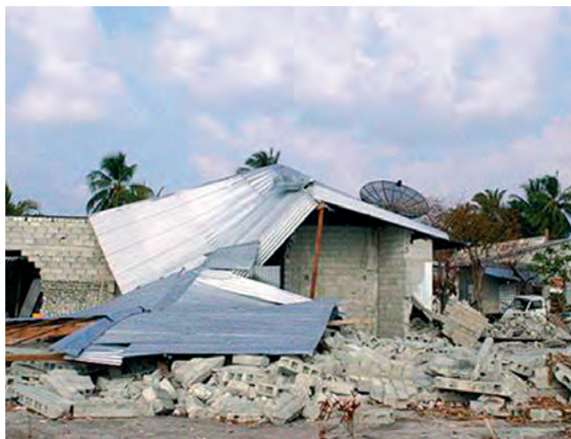
School buildings in the Maldives destroyed by the tsunami of 26 December 2004
