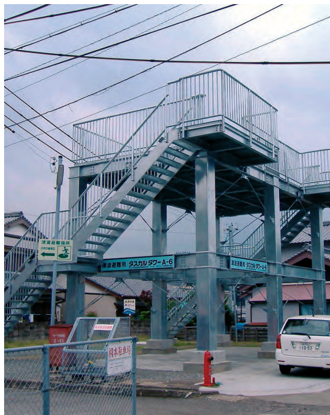
A newly constructed town centre tsunami evacuation tower
