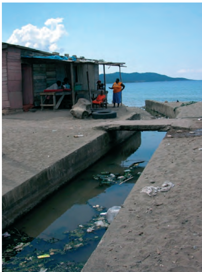
Residents living on the banks of the Mother Ford. This drain is frequently blocked by sand bars deposited by the sea, which residents have to clear to prevent flooding of adjacent homes
